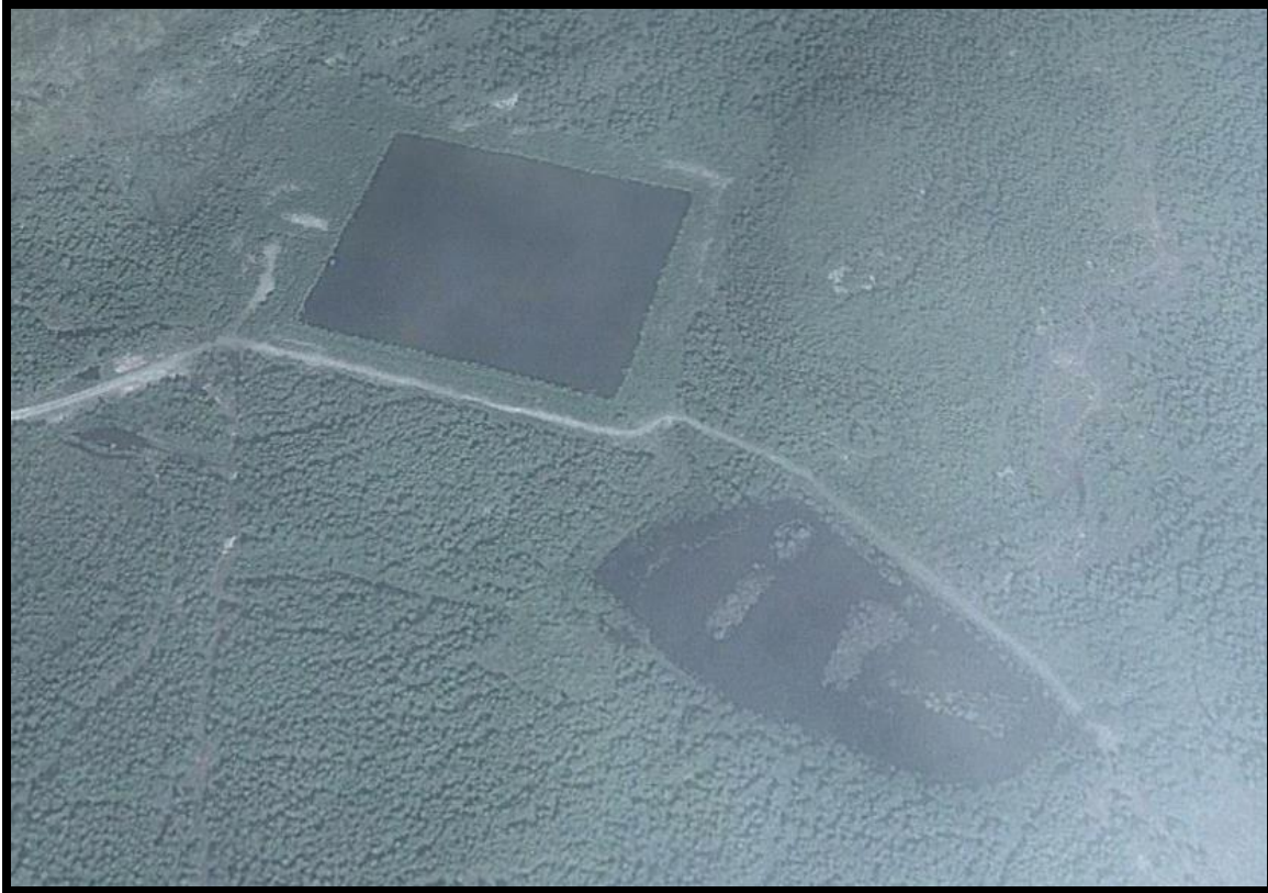
Figure 10 - Aerial Photo of the Benton (Constructed Wetland) Management Unit
